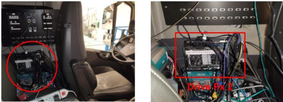
Figure 34: Inference hardware installation in the Golden Truck.
